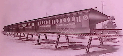
As a train of the Valentine Mono-Railway System will appear, each car a complete unit. Average speed upwards of 150 miles an hour in absolute safety.
