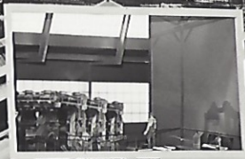
A SHEET MILL. SHEETS ARE ROLLED TO REQUIRED THICKNESS FROM SLABS OR CAKES
