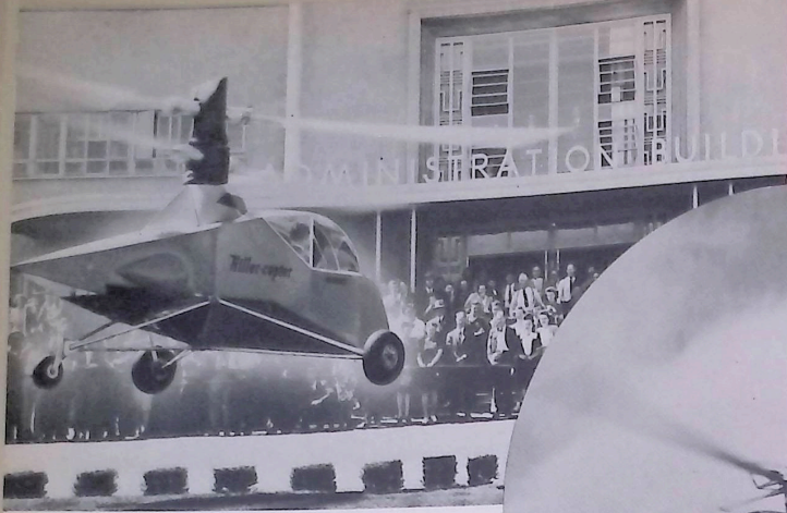
PHOTOGRAPH COURTESY KAISER CARGO, INC.
