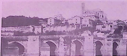
St-Pierre's bridge, at Limoges.
