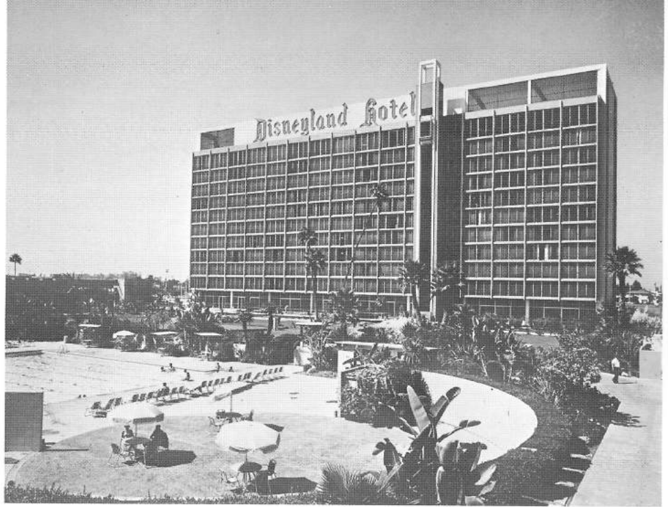
Construction of a new Disneyland Hotel tower, much like this one, will begin this Spring, increasing guest capacity by 50 per cent. The new tower will stand to the right of the present one and face north.
