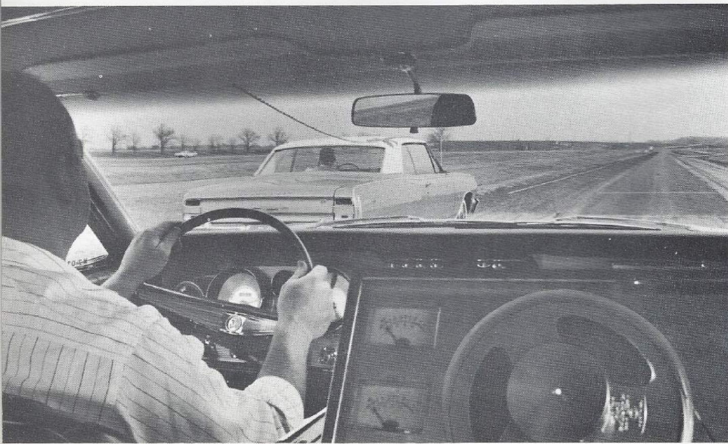
Chevrolet Chevelle “wired for sound” drives on rough-textured road at Milford Proving Ground. Cable carries road noise to instruments in laboratory car
