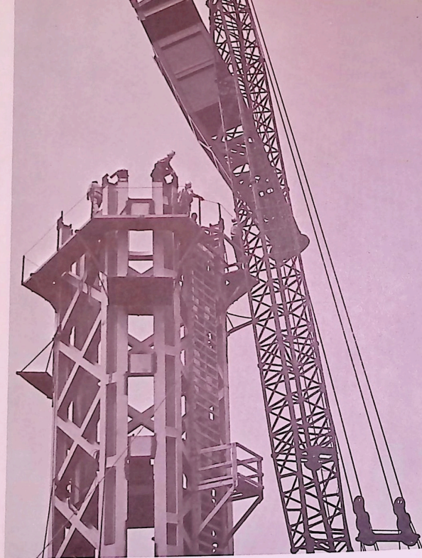
Part of self-contained Space Needle derrick goes into place on 68-foot-high core.
