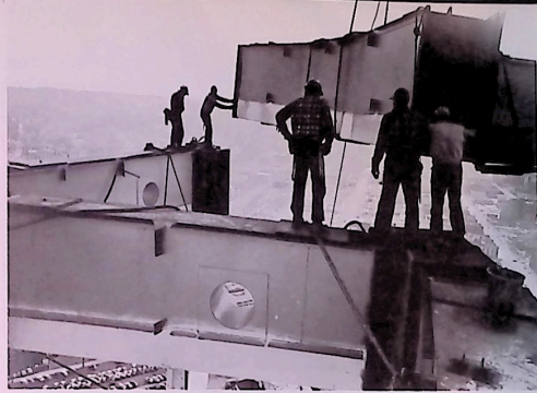
Steady nerves on top bring ring girder section to its berth.
