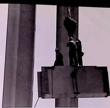
They "ride the iron" when there's no other way to get there. This is box beam to unite a pair of legs.
