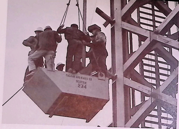
"Sky, please." Seven men in a "skip" full of steel are crane-borne to work.
