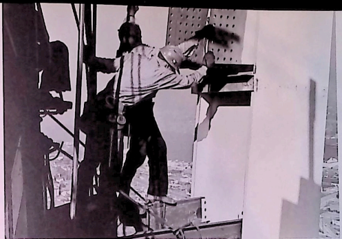
Two men now wrestle with it, man behind beckoning skyward to crane signalman. Bent "spud wrench" in hand bespeaks struggle.
