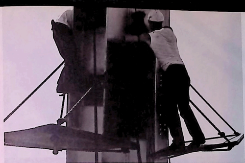
"Float" riggers shimmy up their limbless tree to provide dizzy security for bolters who will follow.
