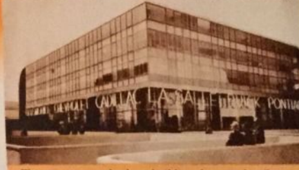
This copper and glass building houses the Automobile Display Salon where cut-away chassis and engines explain details of automotive construction.
