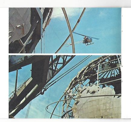
steel orbit rings that circle Unisphere are anchored by thin stainless steel aircraft cable, barely visible from the ground.
