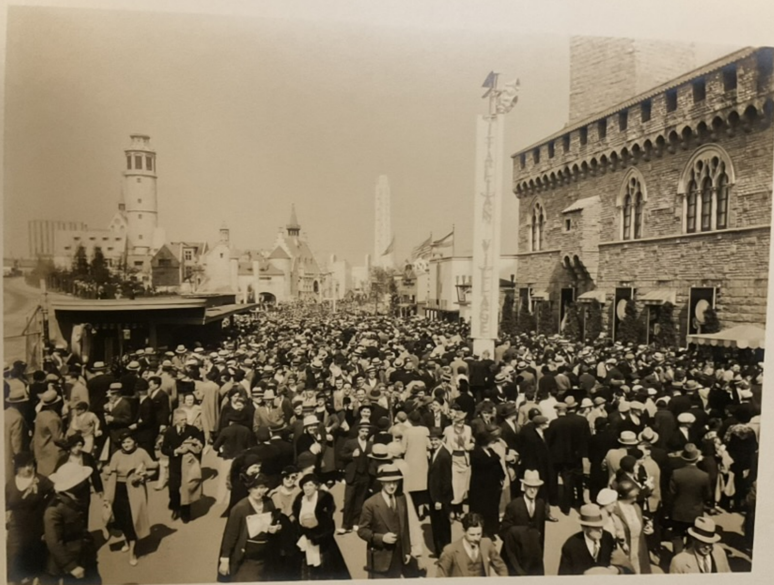
Village Area - looking North
