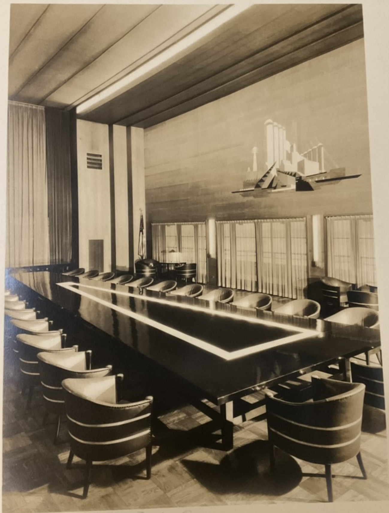
Administration Bldg. - Trustees Room
