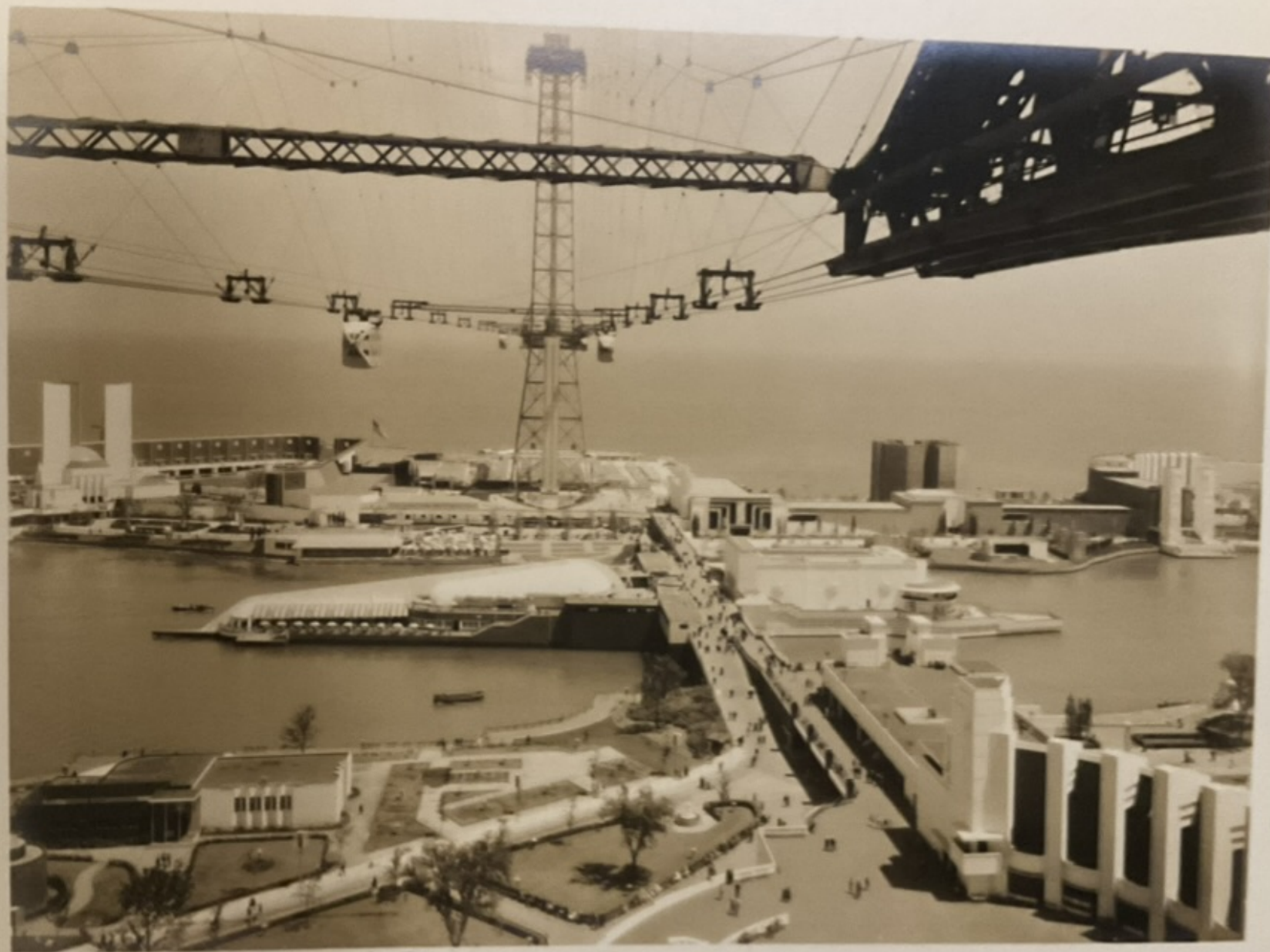
Looking East from West Hydrant Tower
