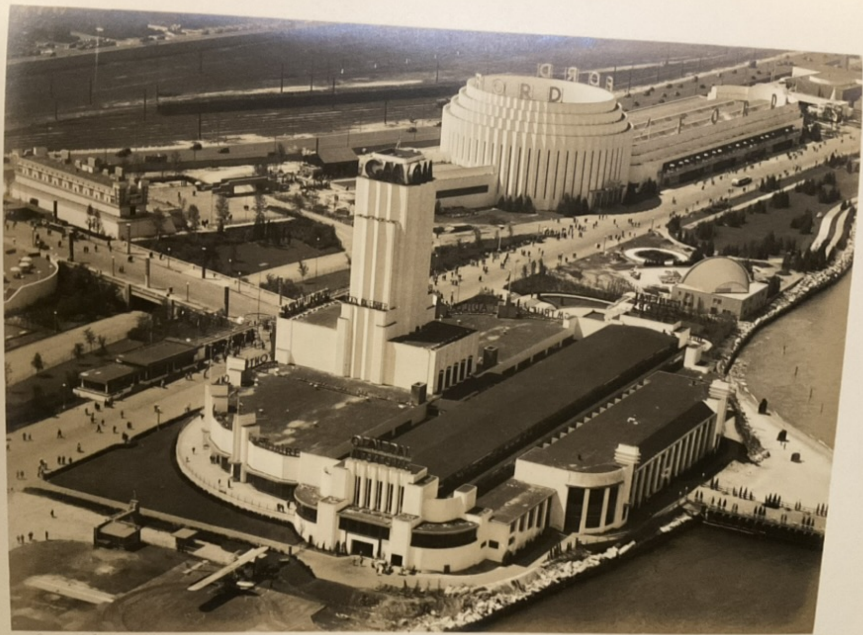
Aerial View at 31st Street
