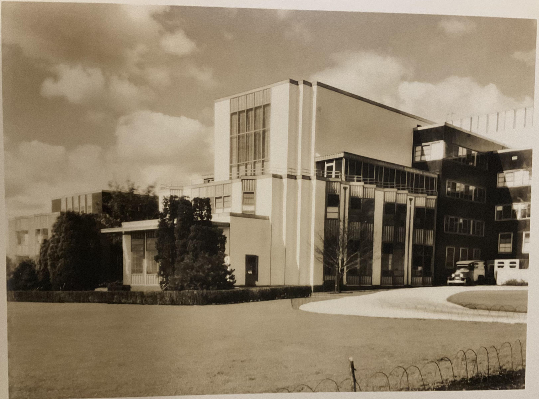
Administration Bldg. East Facade
