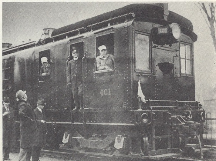
This was the granddaddy of all diesel locomotives. Old No. 401, shown on one of its experimental runs in 1926, was the first diesel ever to be used in road service. Many developments worked out on this locomotive are standard on today's modern diesels.
