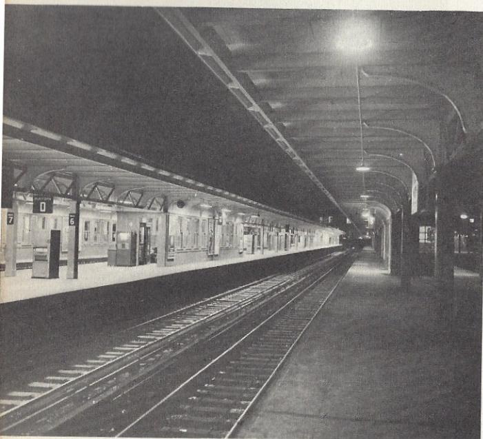
The new and the old in today's modernization is vividly portrayed in this photo of the Jamaica Station while the job of installing new fluorescent lighting was under way in 1958. Spotty, dim lighting of old lamps on one platform contrasts sharply with the bright, even illumination of the fluorescents on the other. Jamaica is now one of the most brightly lighted stations in the Nation.
