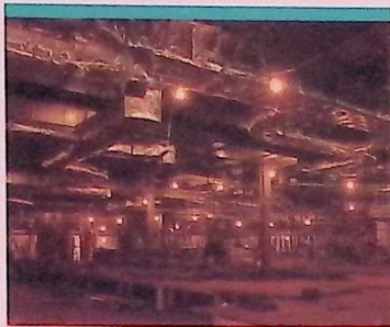
Construction on the Seabase mezzanine was well advanced by May of 1985.
