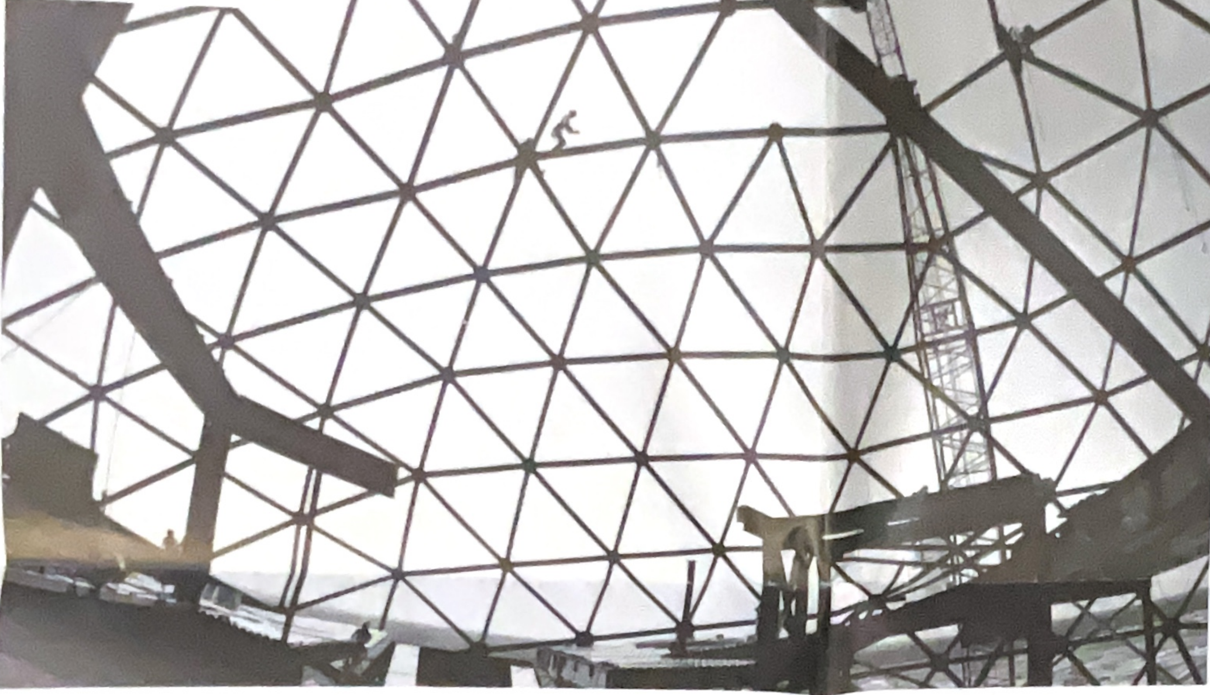
Steel Spiderweb — Spaceship Earth, the 180-foot tall Epcot Center landmark, towers over the construction site with geodesic patterns of steel. Several of the nearly 2,000 workers on the job assemble the huge globe.
